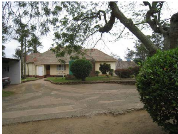
Fig 4: Main house from the south
