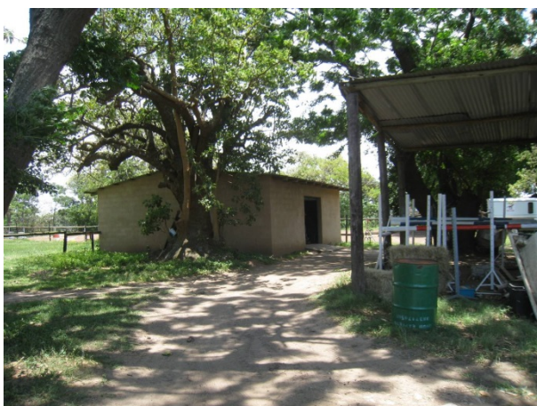
Fig 43: Building 2 from the south
