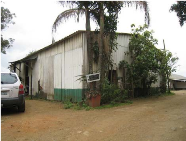
Fig 35: Building 4, wood and iron barn
