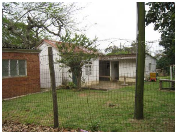
Fig 16: Labourer's cottage rear (east) view
