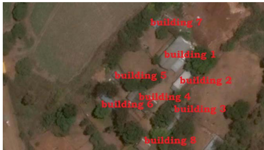
Fig 26: Buildings on site 2 under discussion
