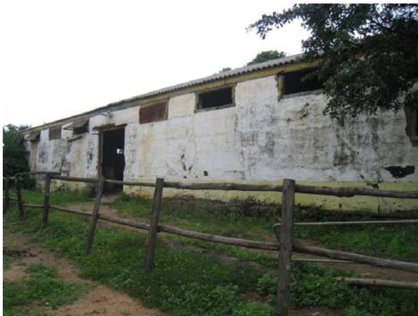
Fig 31: Barn from south west
