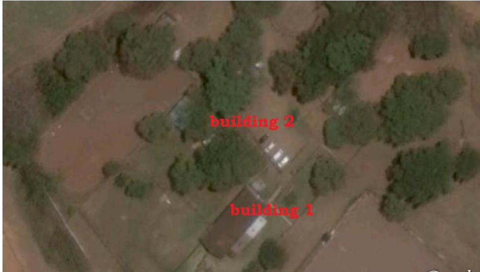
Fig 40: Buildings on site 3 under discussion
