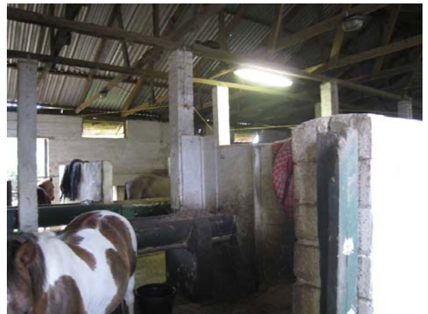
Fig 32: Interior of barn
