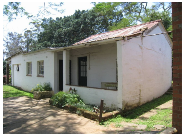
Fig 17: Labourer's cottage, west view
