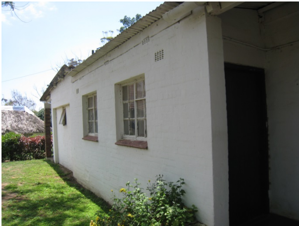
Fig 18: Labourer's cottage extension
