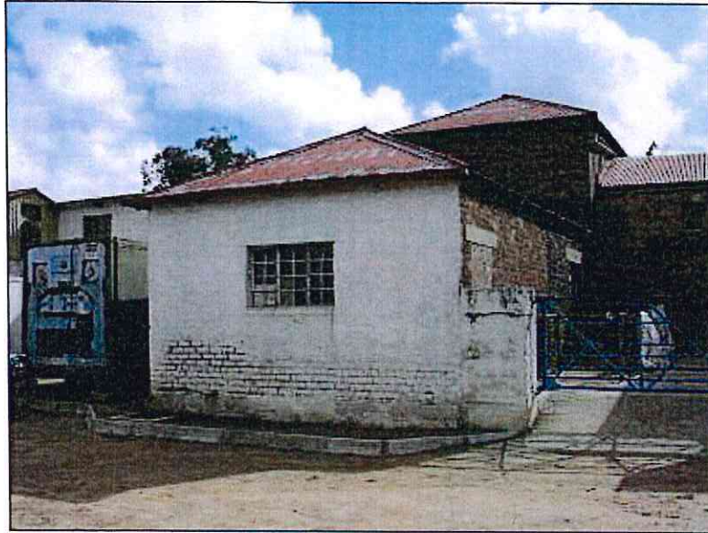
No 5a, front: Small historic building, unknown function No 5d(ii), background: Face brick stores (all to be preserved)
