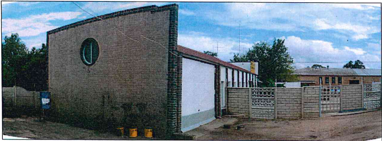
Buildings 5g (left) and 5f (right)
