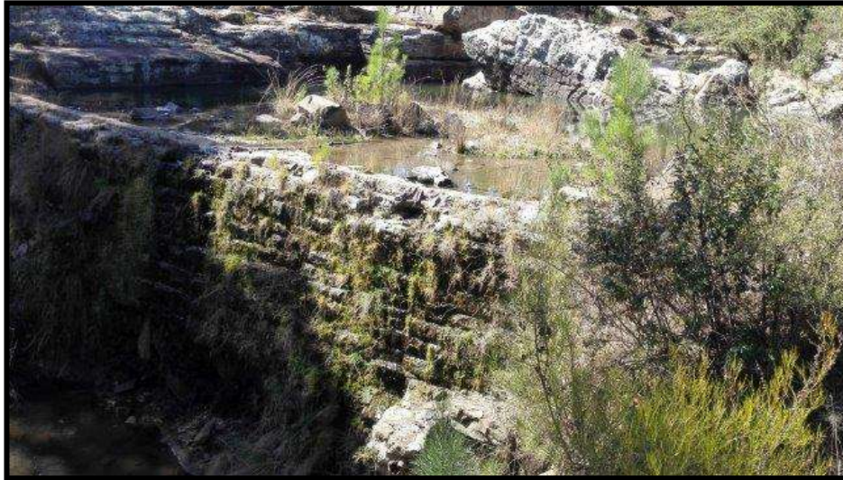
FIG. 7b: BUILT STRUCTURES AT THE HOGSETT DAM
