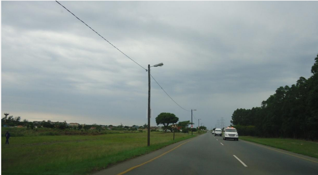
Image of road to upgraded
