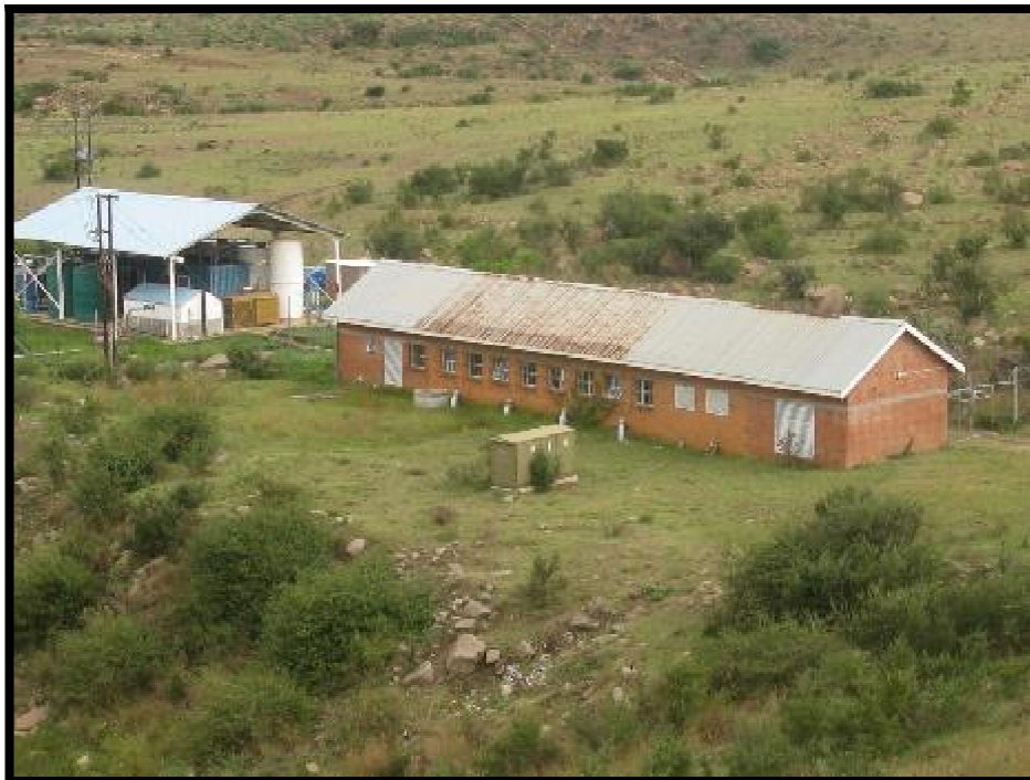
Figure 10. Mvunayane Dam Pump Station.
