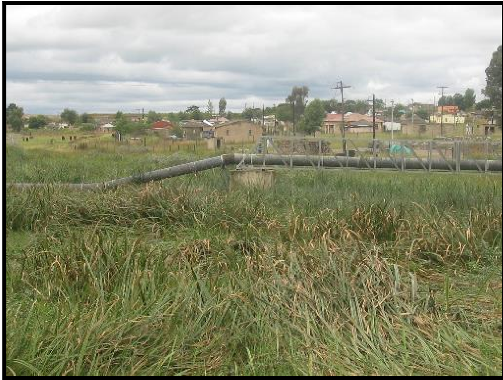
Figure 5. Exposed section of the 4km replacement pipeline.
