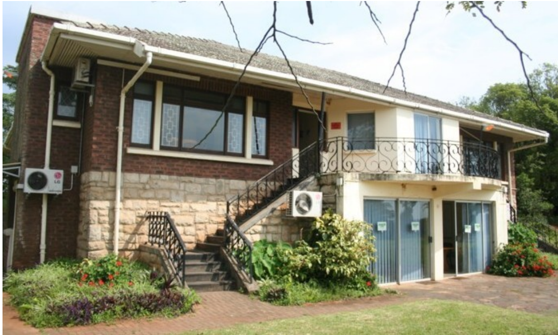
Fig 2: Affected structure on Lot 91 Umlalazi (photo: supplied)
