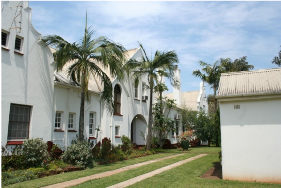
Fig 13: Rear view of Highfield Country House (photo: supplied)
