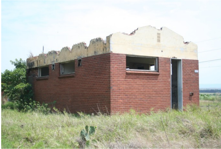
Fig 7: Showing remains of station building (photo: supplied)
