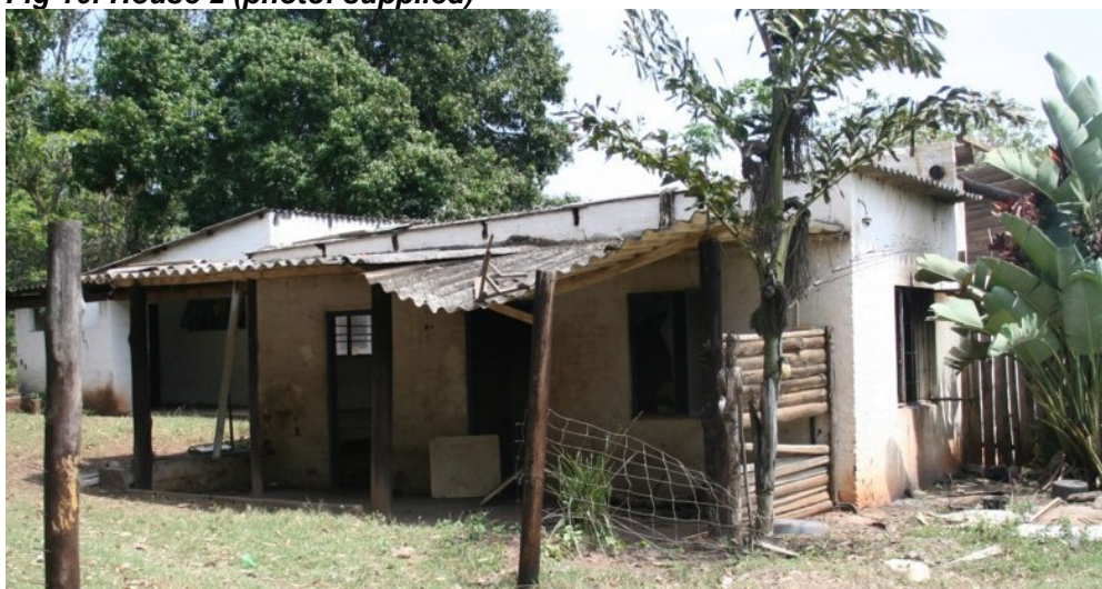
Fig 17: House 2 labourers cottage (photo: supplied)
