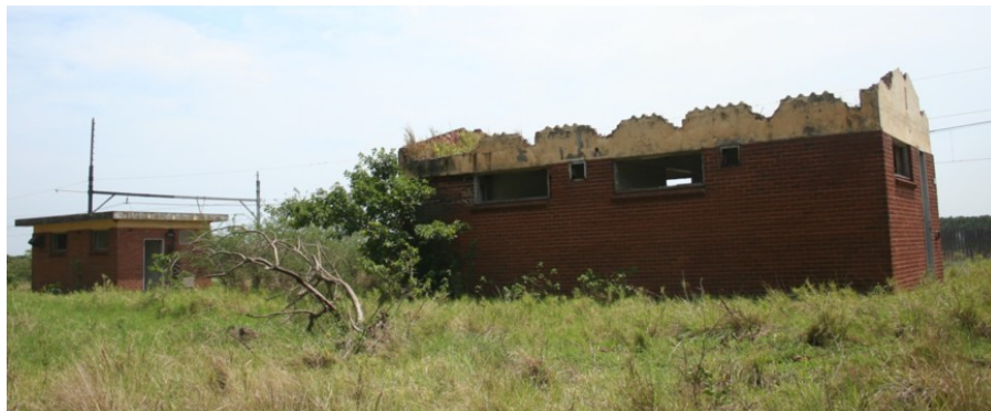
Fig 6: Showing remains of station building (photo: supplied)
