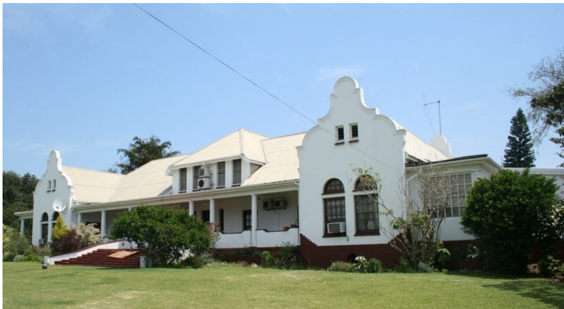
Fig 11: Showing front elevation of Highfield Country House (photo: supplied)
