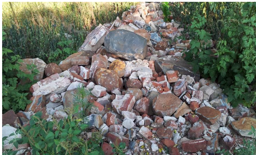
Figure 8: Large heap of building rubble associated with the demolished structure
