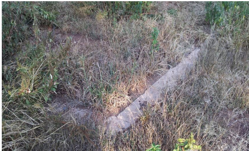
Figure 7: A section of a cement foundation
