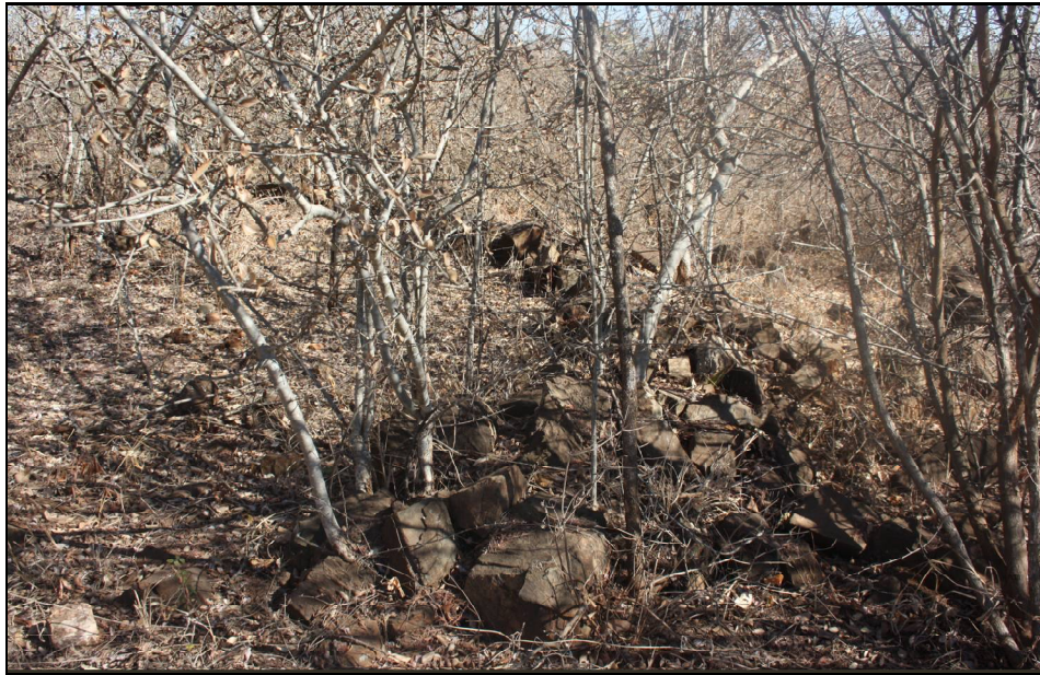
Figure 5: Section of half circular stone wall, which forms part of a homestead (Site No 003)
