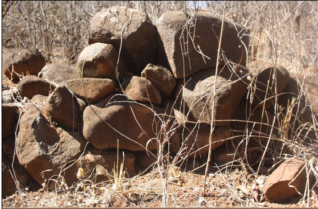
Figure 16: View of the still intact stone wall (Site No 010)
