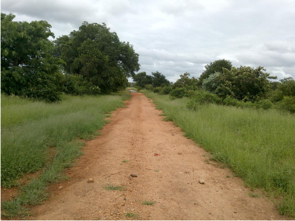
Figure 2: View of the gravel road traverses along the proposed site.
