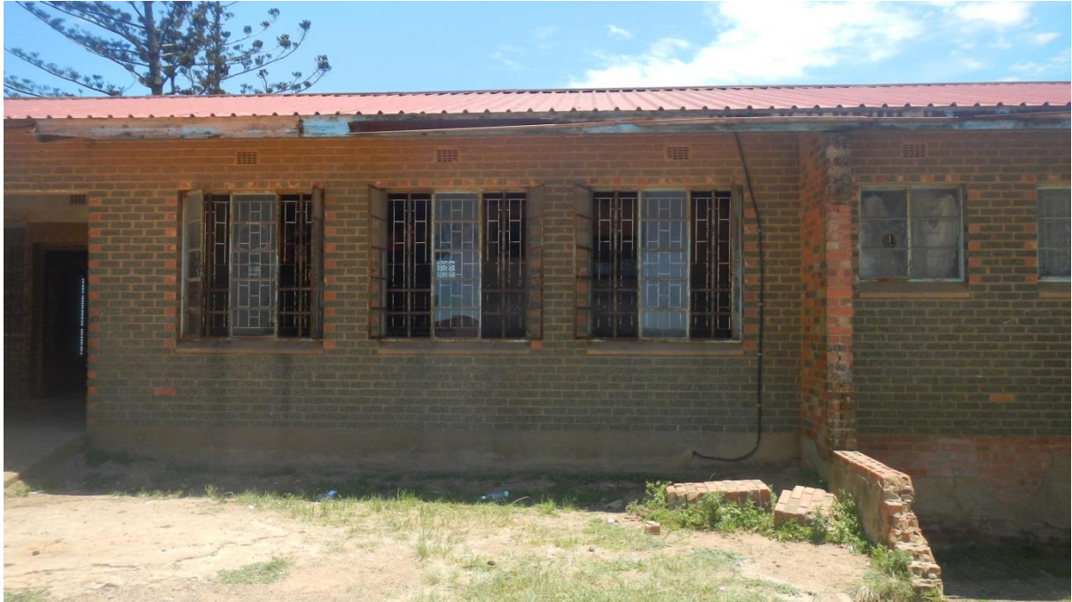
Figure 5 : Front end façade of the post office building block A.
