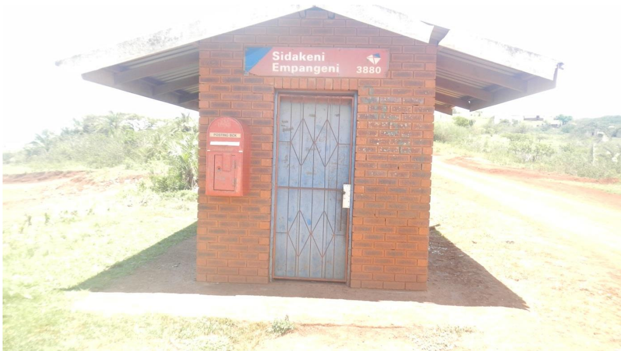
Figure 12: Front façade of the Sidakeni- Empangeni small posting box
