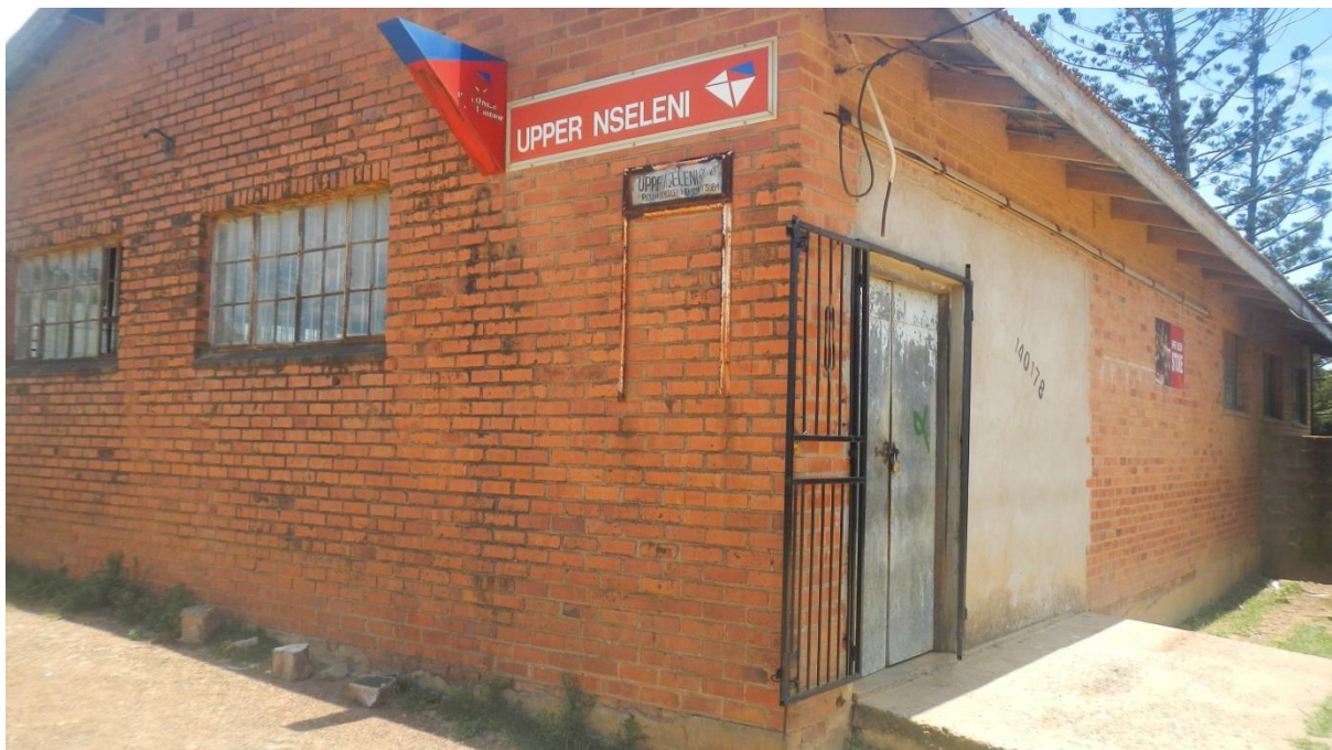
Figure 8: Western view of the second post office block (Block B)
