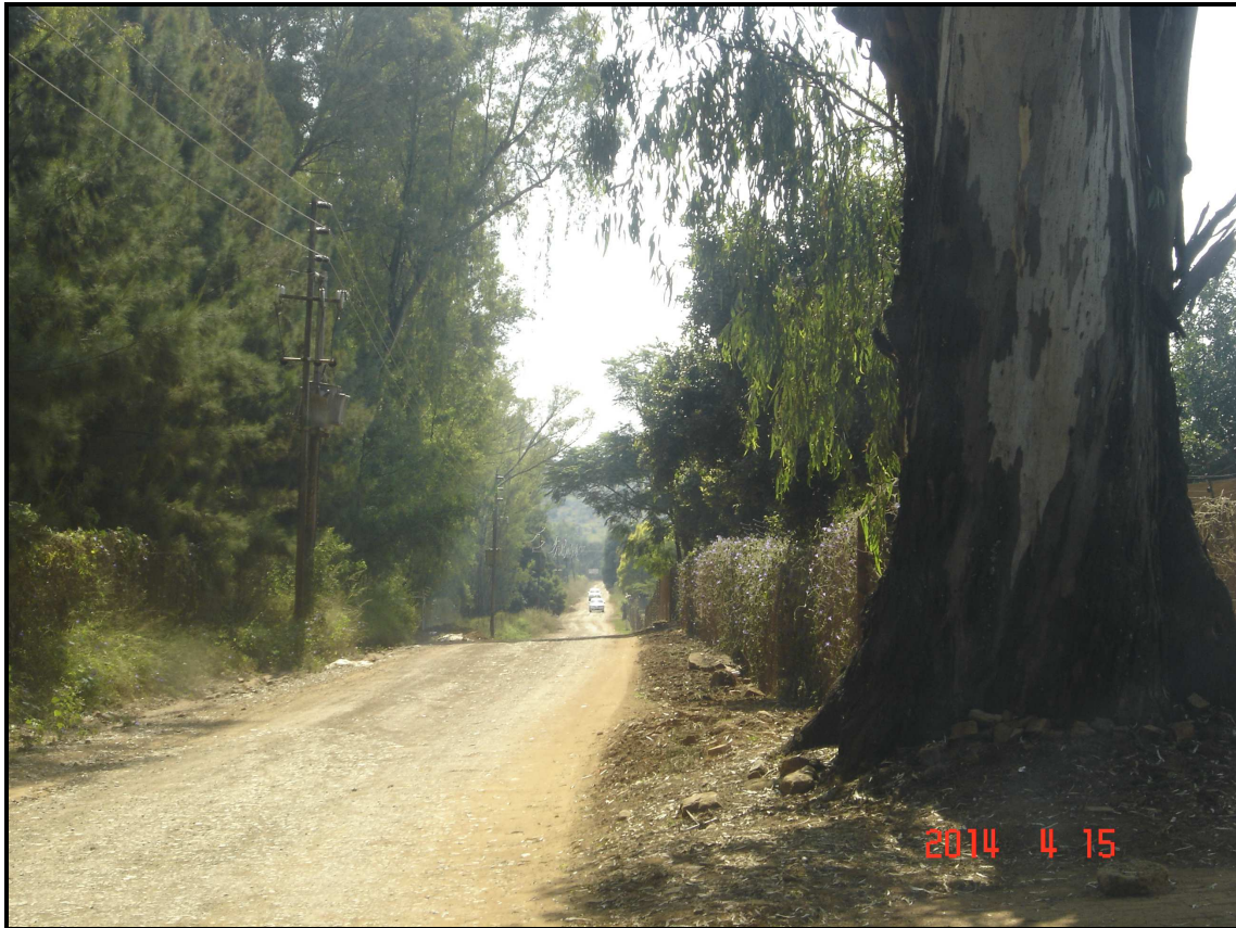
Plate 1: Existing gravel road
