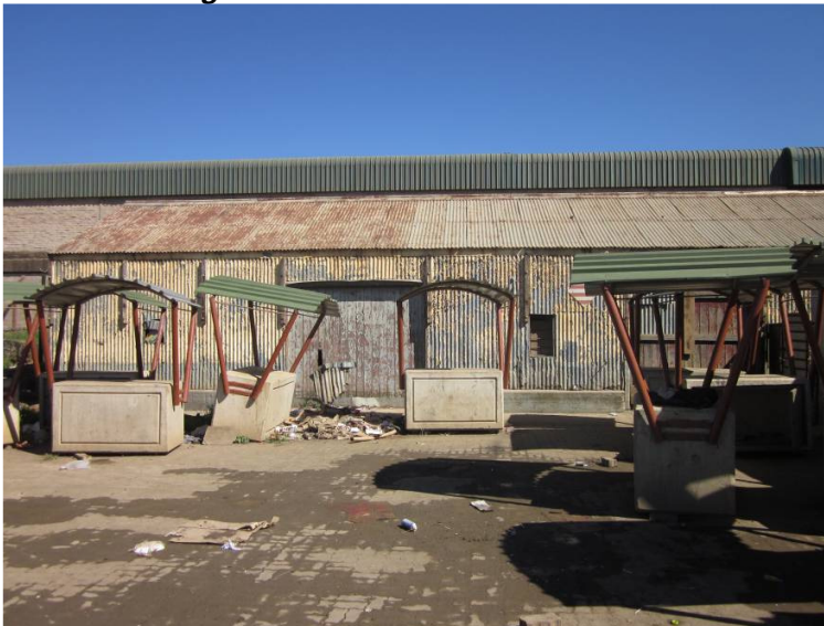
Fig 7: Eastern elevation showing hawkers stands in the foreground
