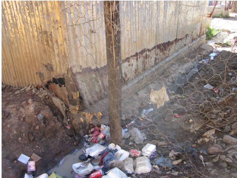
Fig 9: Condition of base of building
