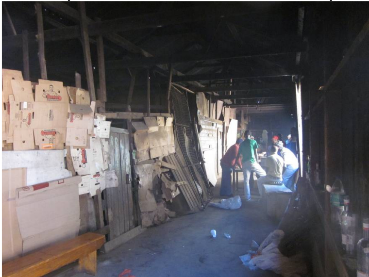
Fig 15: View along the length of the interior of the shed
