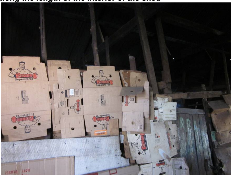
Fig 16: Detail of room dividers inside the shed
