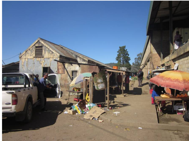
Fig 4: Showing the front elevation, accretions and alterations in roof pitch
