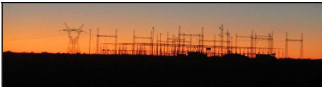
Figure 49: Evening view of the large Eskom substation located some 16 km south of the proposed project.
