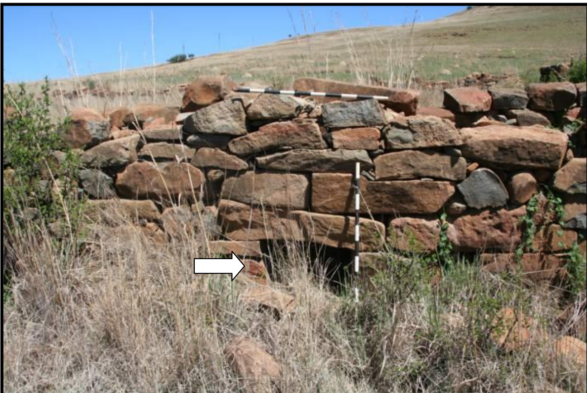
FIG. 12: DRAINAGE HOLES ALONG NORTH WALL
