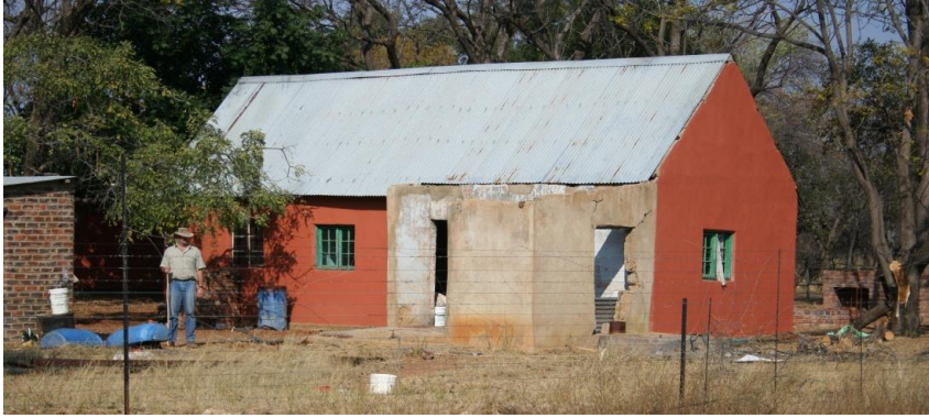
Figure 5.6. Brick building on Ringbult: CB15 .
