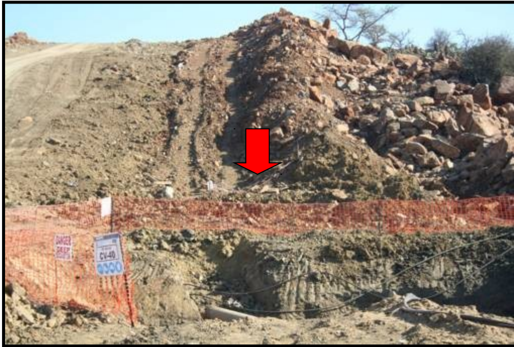
FIG. 22: BACKFILLING AFTER THE AREA HAD BEEN CLOSED 8
