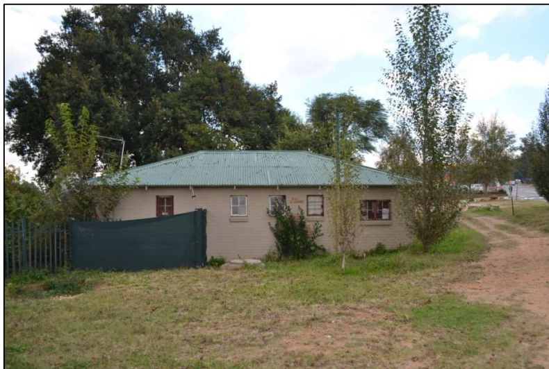
Figure 4. North western elevation of the restaurant building
