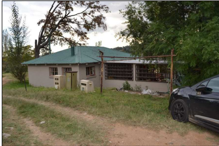
Figure 3. Southern elevation and view from Centenary Street towards the restaurant.
