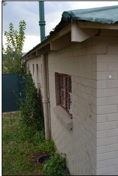
Figure 5. The unplastered but painted exterior of the building
