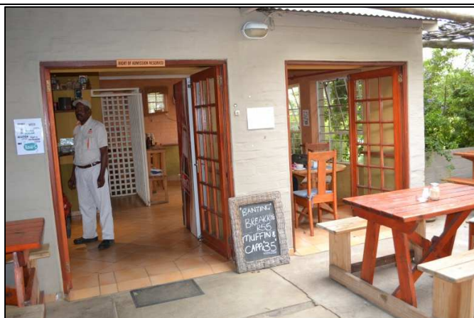
Figure 7. Timber frame double doors installed to allow free movement from the interior to the patio.
