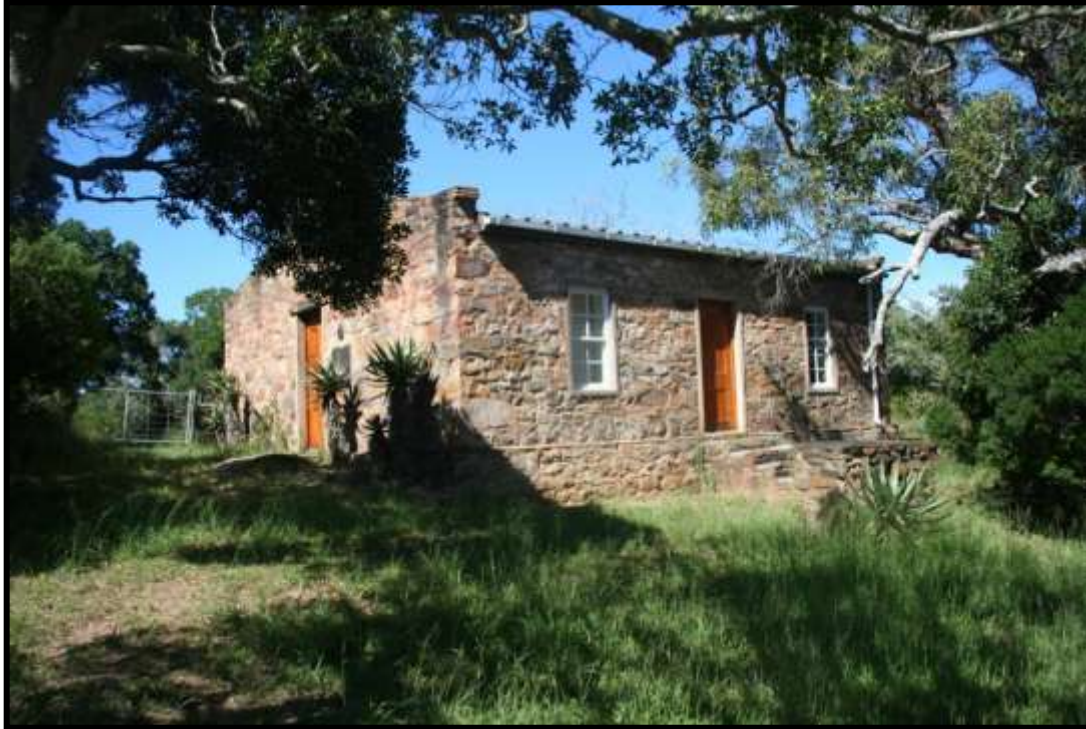
FIG. 31: BUILDINGS AT CUYLERVILLE CHURCH
