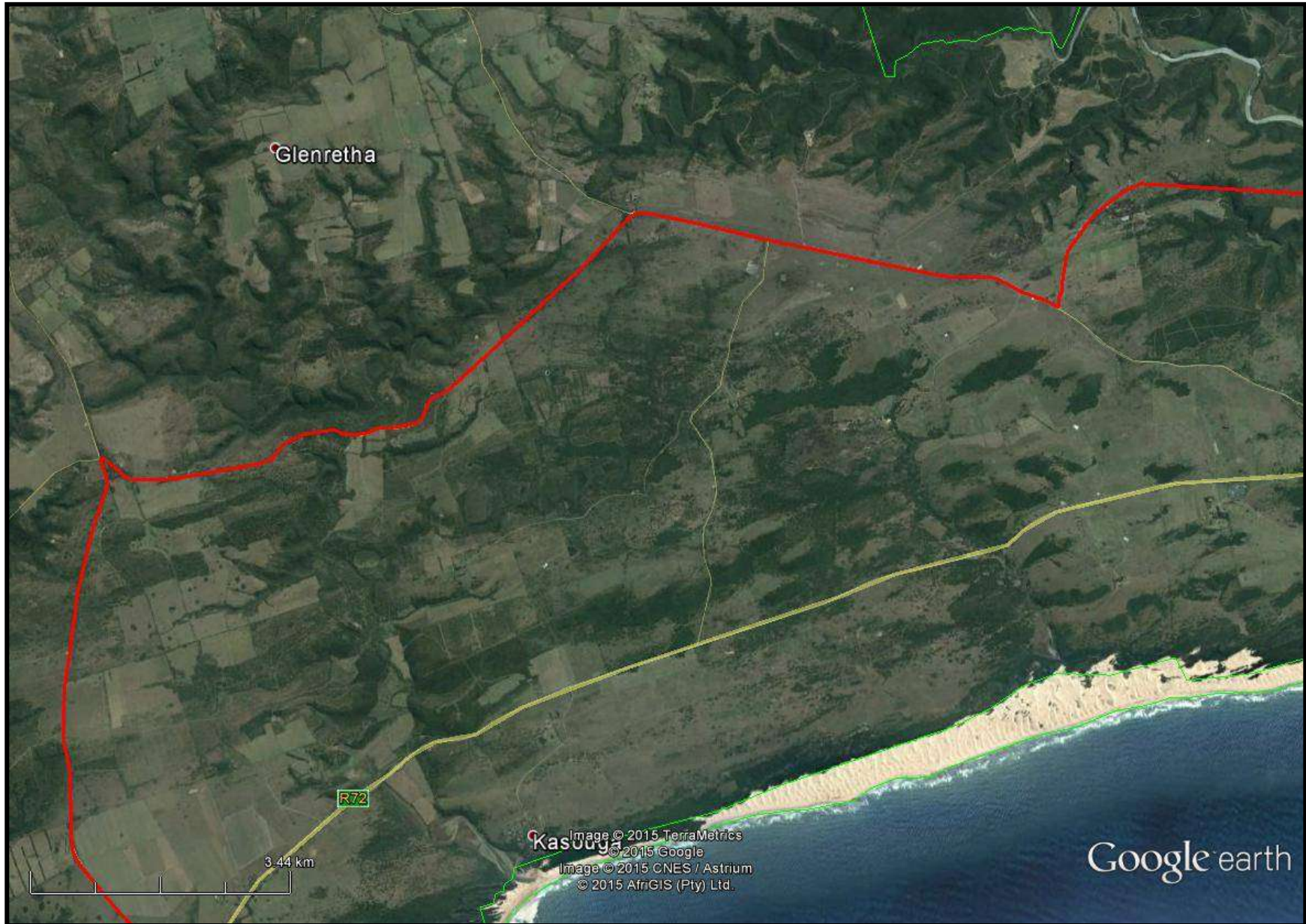
FIG. 2B: AERIAL OVERVIEW OF THE NDLAMBE PIPELINE
