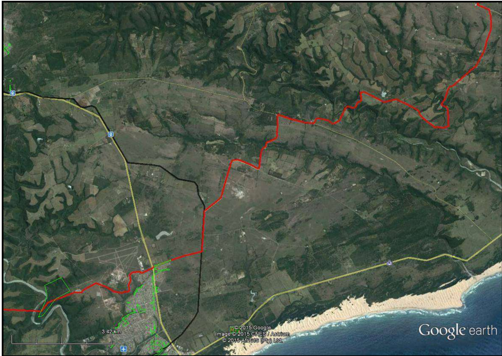
FIG. 2C: AERIAL OVERVIEW OF THE NDLAMBE PIPELINE
