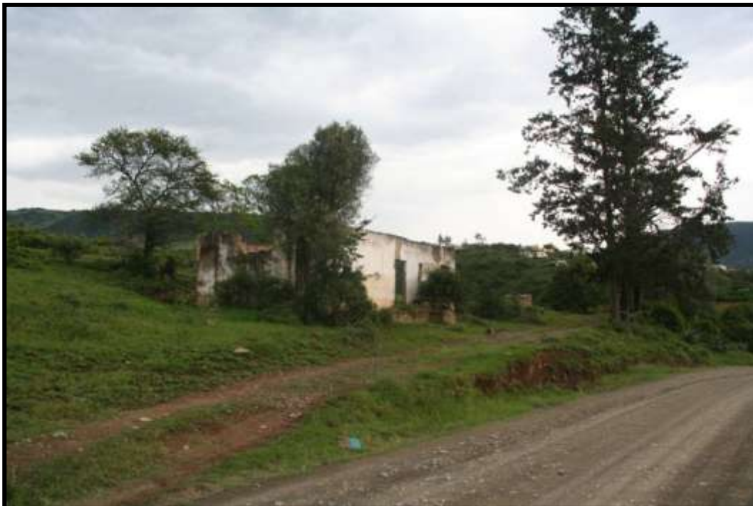
FIG. 7: BUILDINGS AT AMA02
