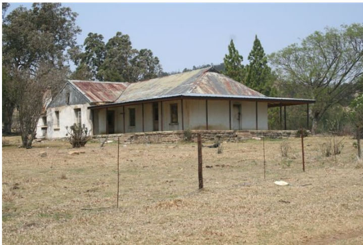
Fig 1: Front view of house, showing suspected later extension
