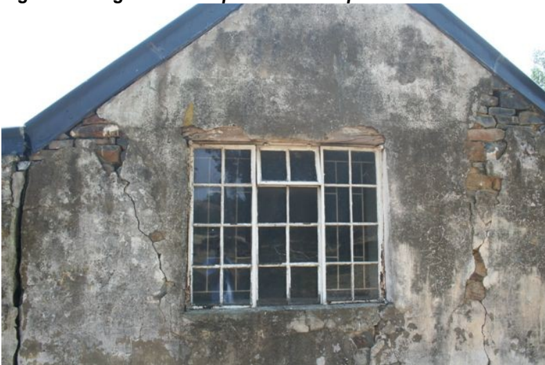
Fig 4: Showing suspected early part of house and inappropriate addition of steel windows
