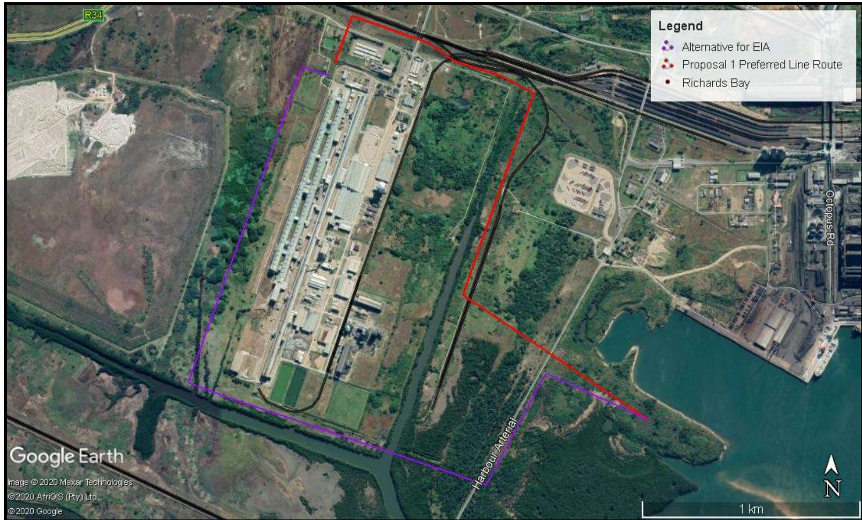
FIG. 2: AERIAL OVERVIEW OF THE PROPOSED DEVELOPMENT
