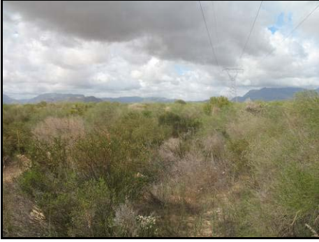
Fig 4. Verlore Switching Station facing north
