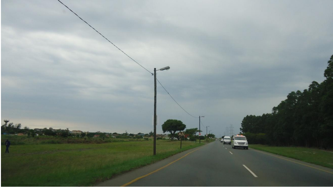
Road to be upgraded, note drainage line
