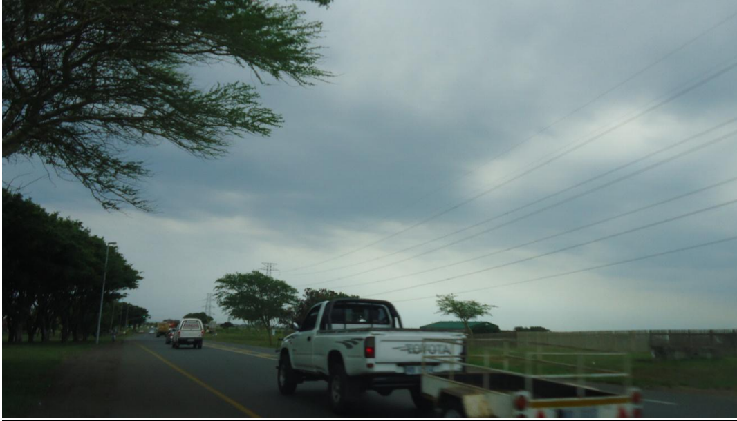
Road to be upgrade
