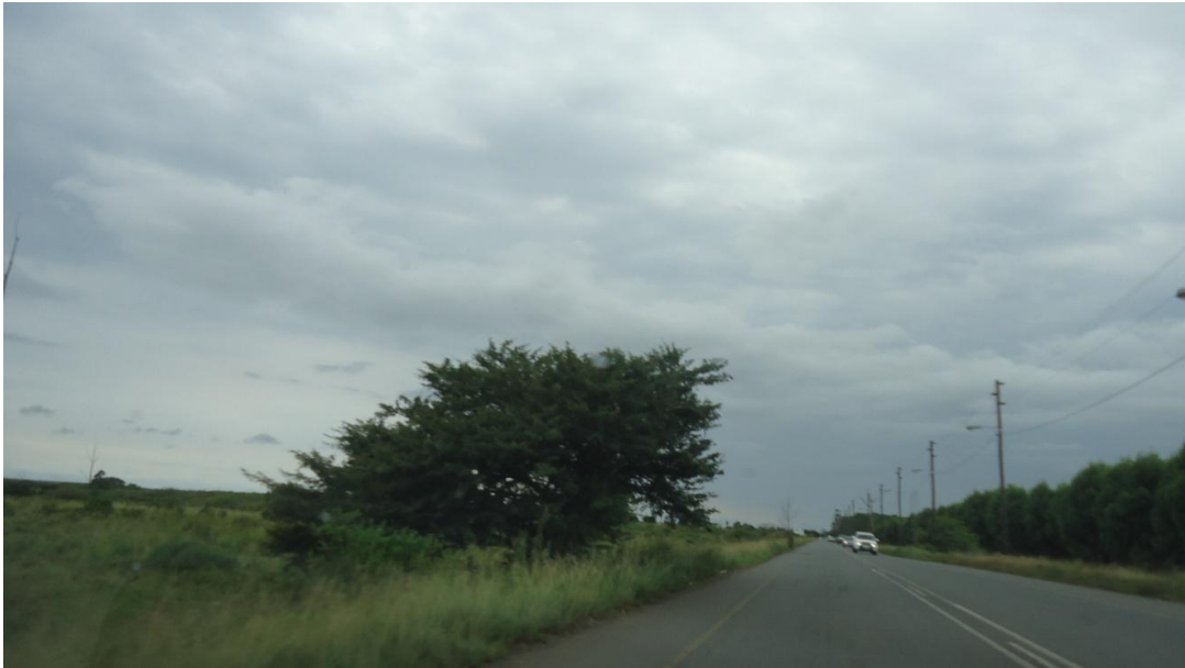
Road to be upgraded
