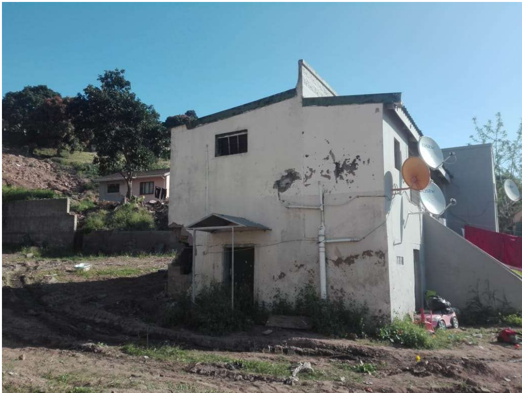
Figure 5: View looking at side of building
