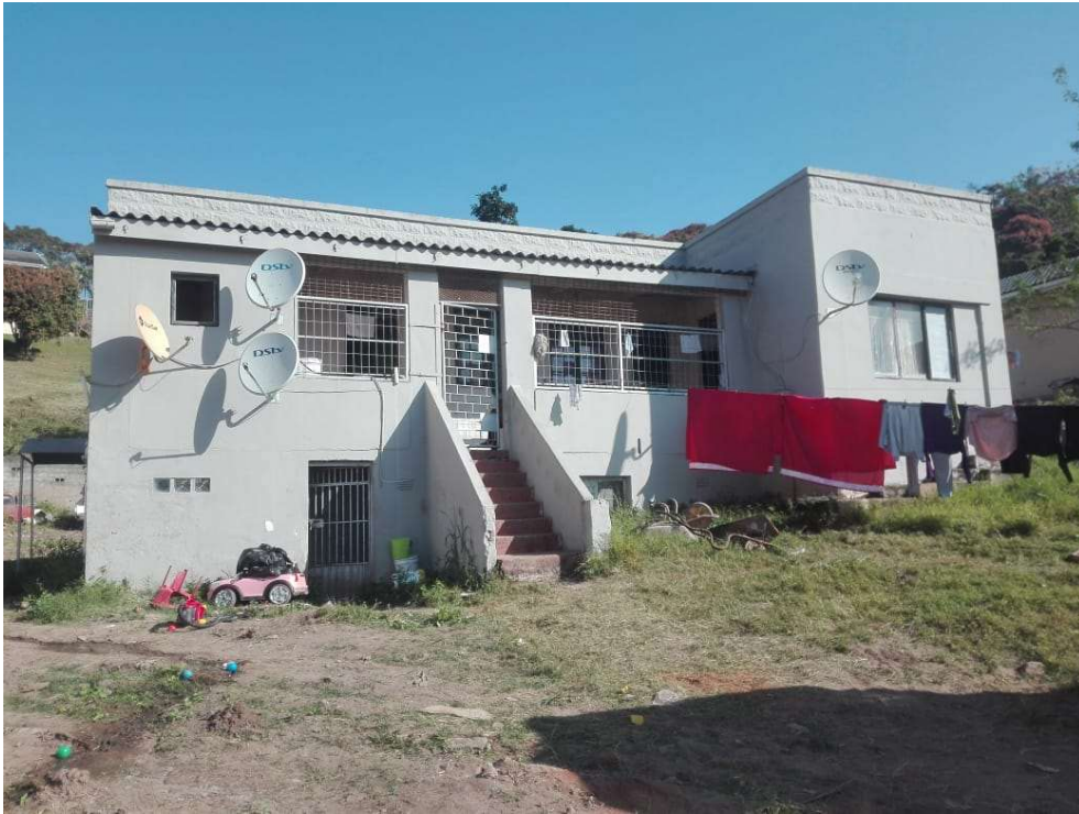
Figure 4: VIEW LOOKING INTO PROPERTY
