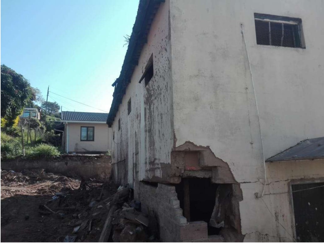
Figure 6: View looking at side and rear of building
