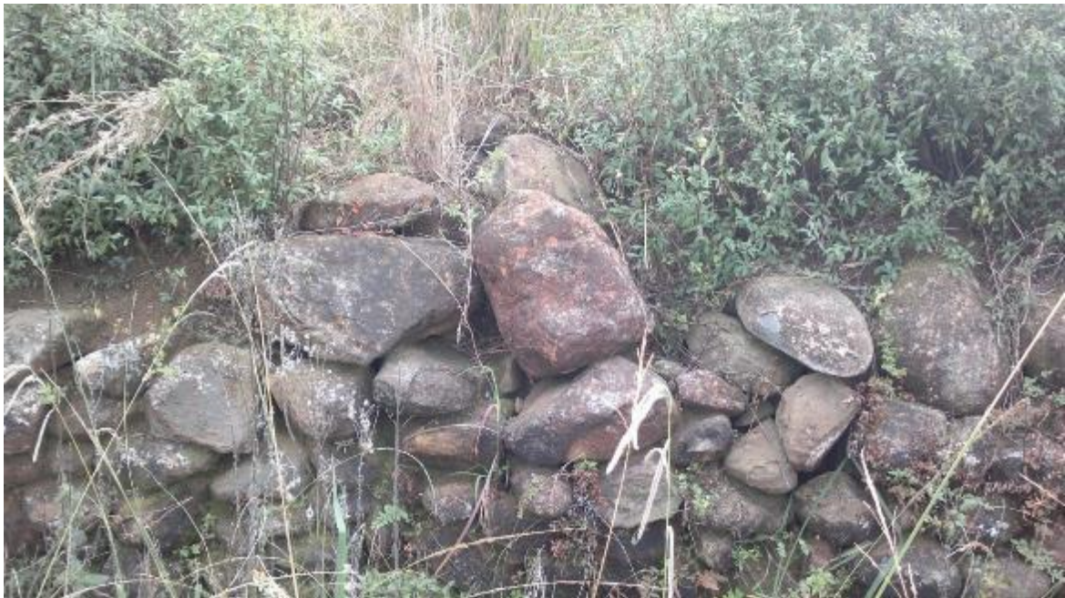
Figure 11: Section of drystone wall
