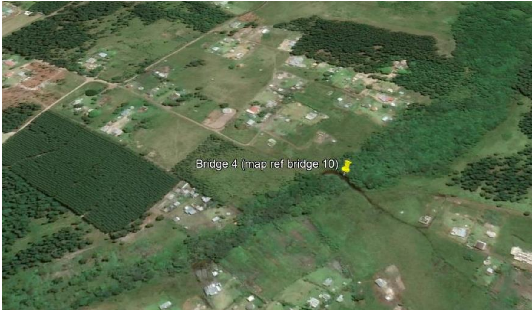
Figure 2: Closer view of bridge No. 10 and surrounds
