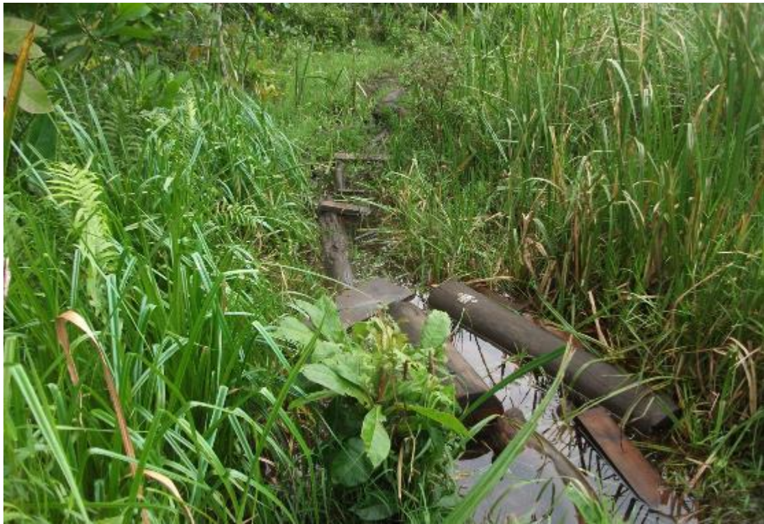
Figure 13: Water clogged northern end of stream crossing
