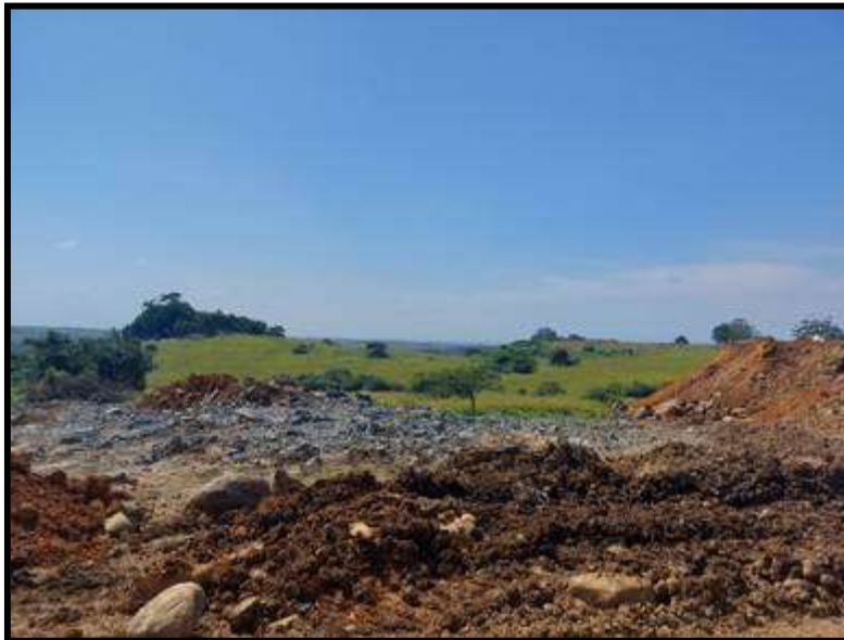
FIG. 11: EARTHWORKS AT THE DEVELOPMENT SITE
