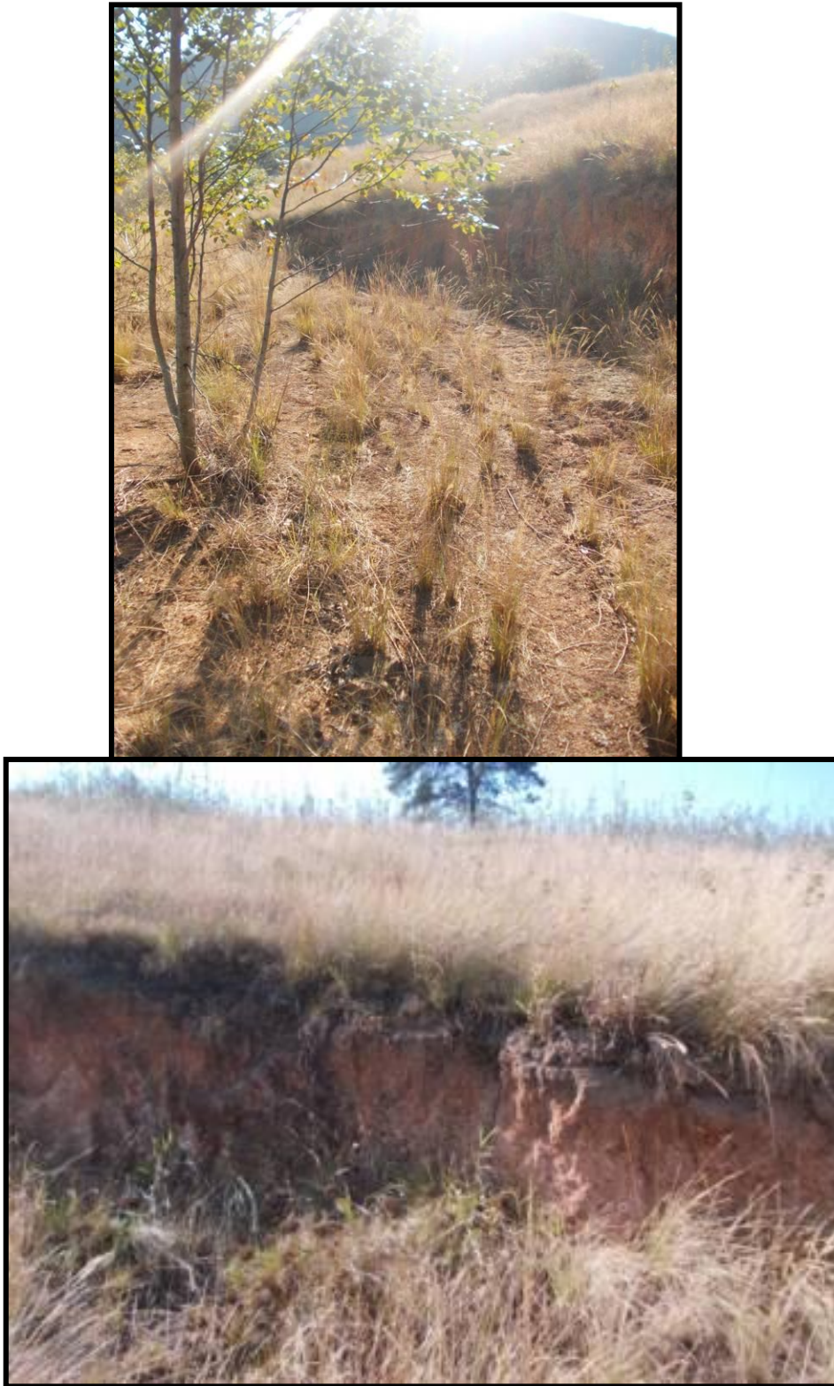
FIG. 9: EXISTING ROAD CUTTING
