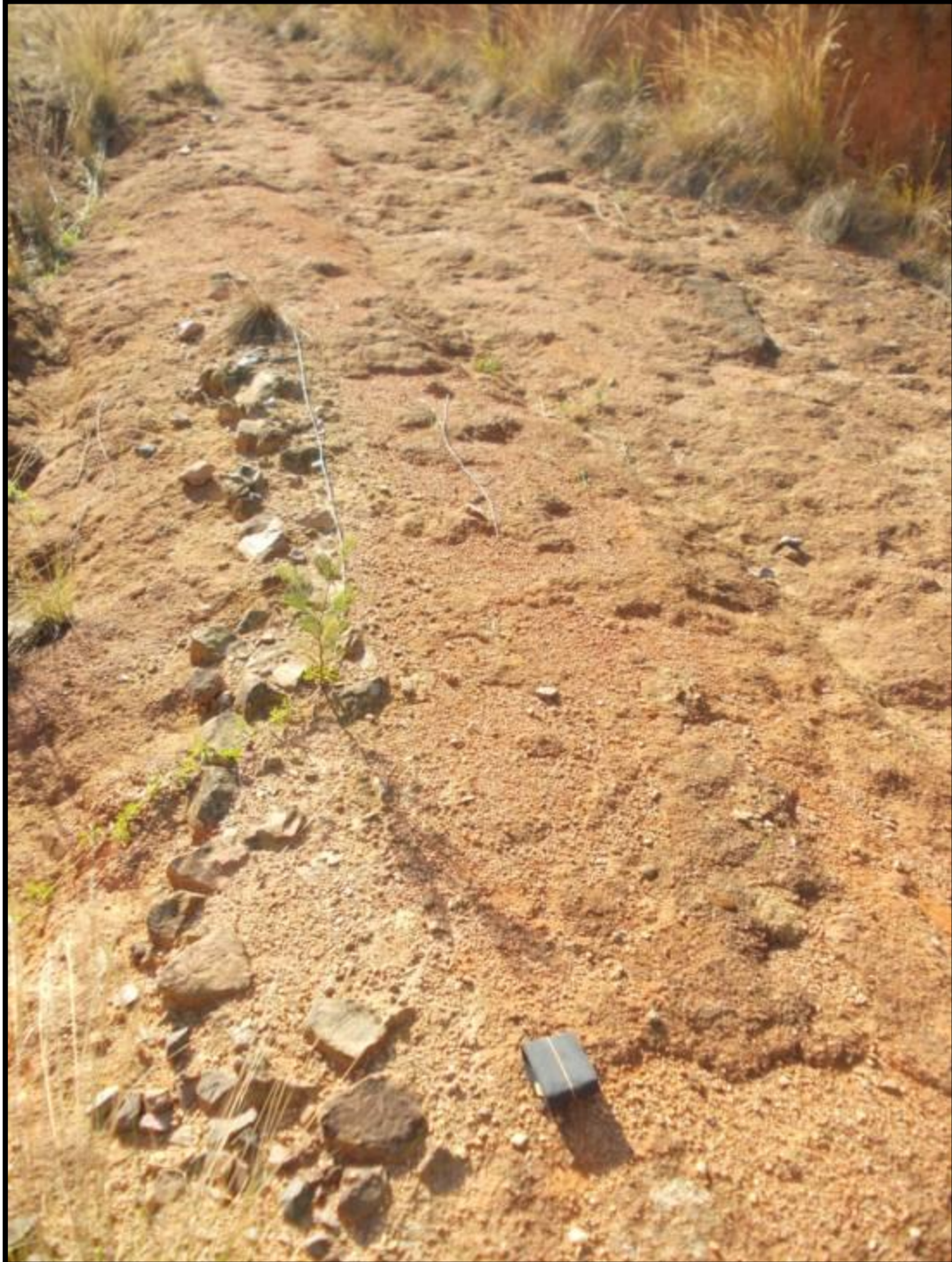
FIG. 10: ROAD "REPAIRS" ALONG EXISTING ROAD AT PATH 1
