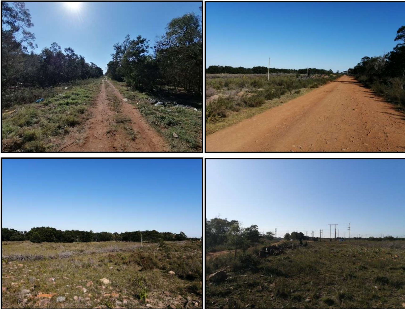
FIG. 4: SCENIC VIEWS OF THE TRANSMISSION LINE
