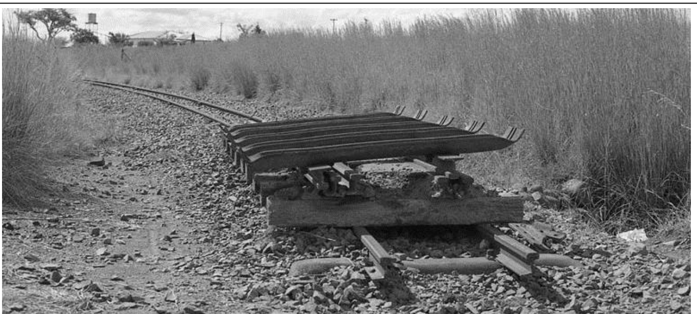
The line was severed for good once the rails were pulled up from the unguarded level crossing over the old Durban – Johannesburg R103 main road, about 6km north of Estcourt, and at the level crossing at Mielietuin – this occurred sometime during 1984. Photo: Bruno Martin
