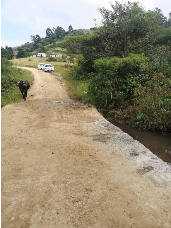
FIGURE 1: STATUS QUO OF THE MBECUKA BRIDGE
