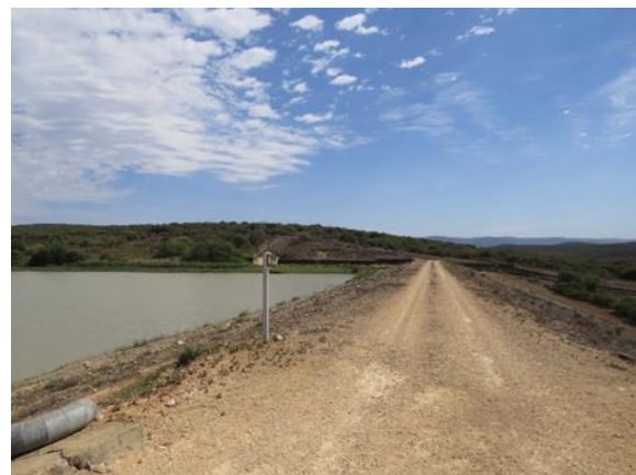
Figure 11: Existing Scheepersvlakte Dam
