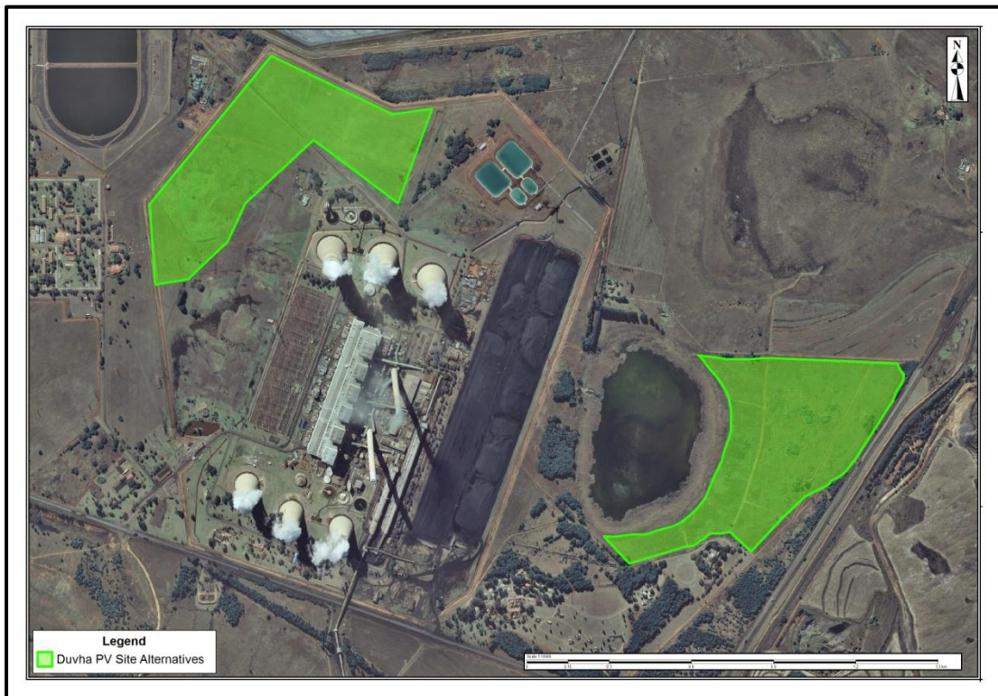
Fig. 5. Location of the surveyed in relation to the power station.
