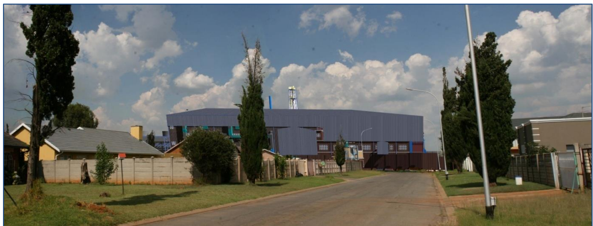
View East from Mey St, without planting, integrated roof structure – proposed expansion
