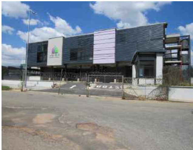
Photo 3 – Existing Areyeng building Adjacent to site
