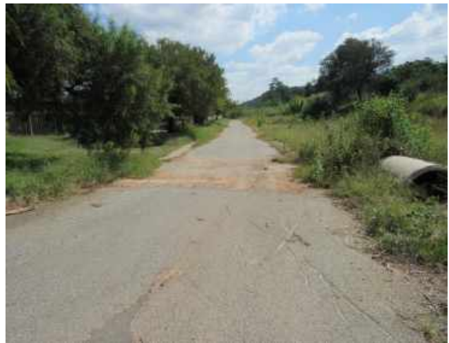
Photo 2 – Existing paved road adjacent to site
