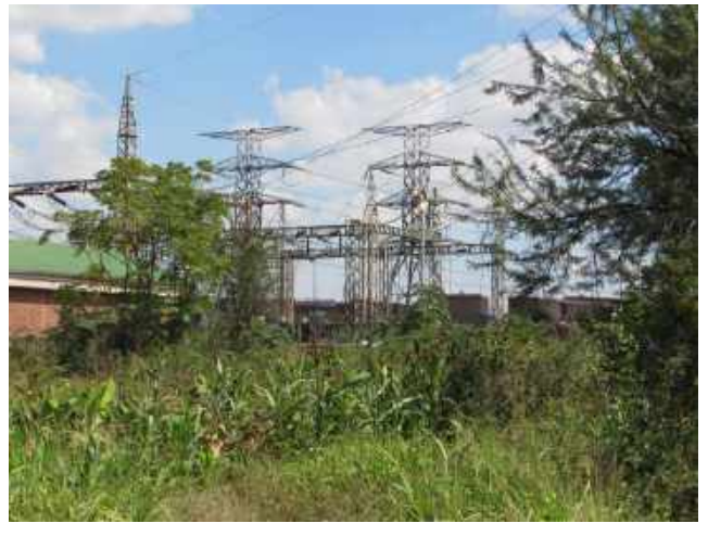
Photo 4 – Existing Power Lines Adjacent to Site
