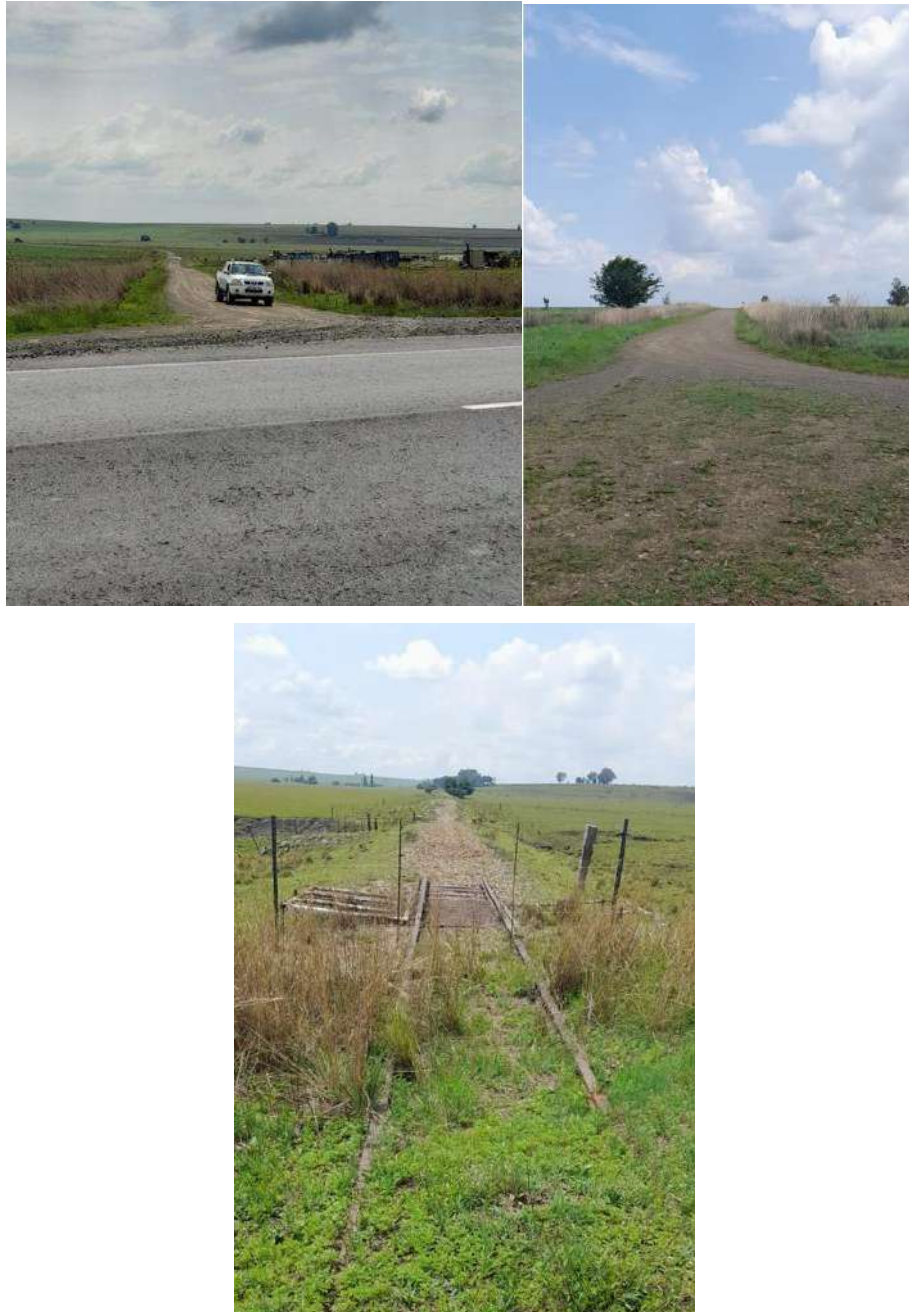
Figure 33: Infrastructure on site.
