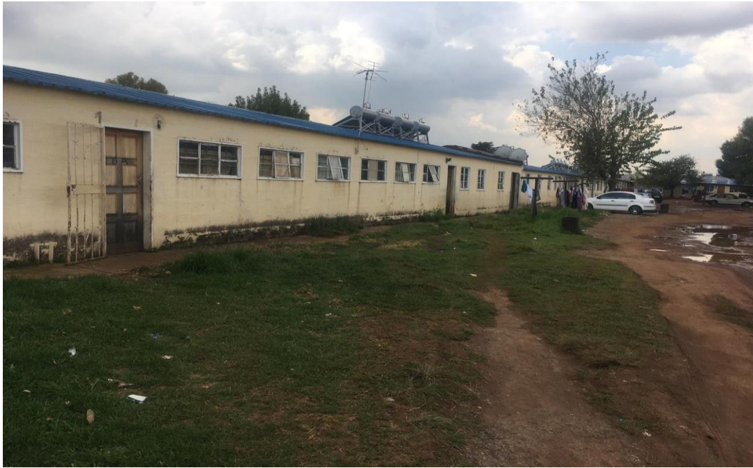
Figure 5 : View of the single quarters hostels at the main entrance from Heald street
