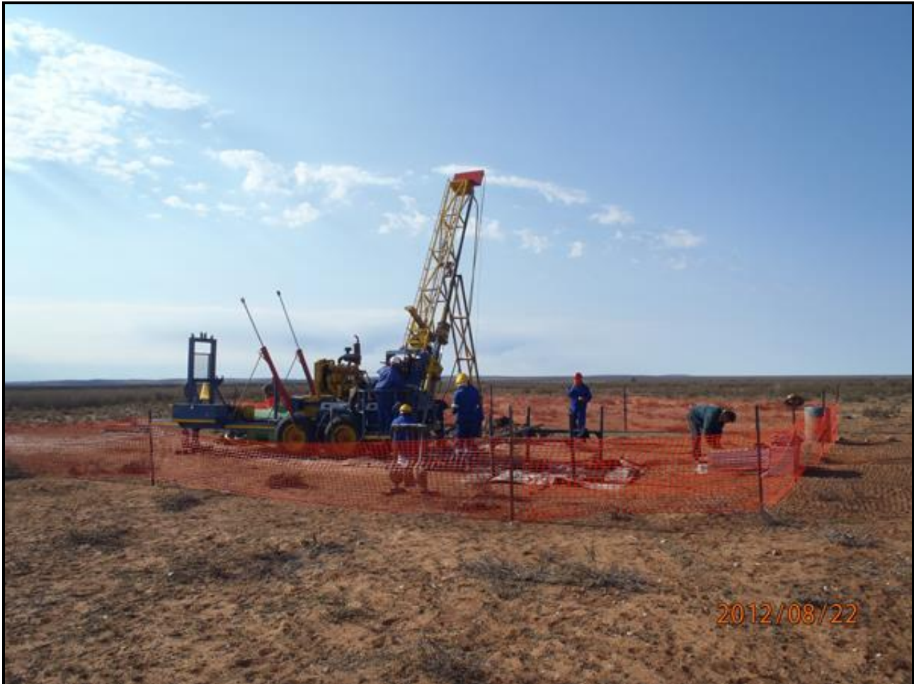
Figure 4: Typical Drilling site
