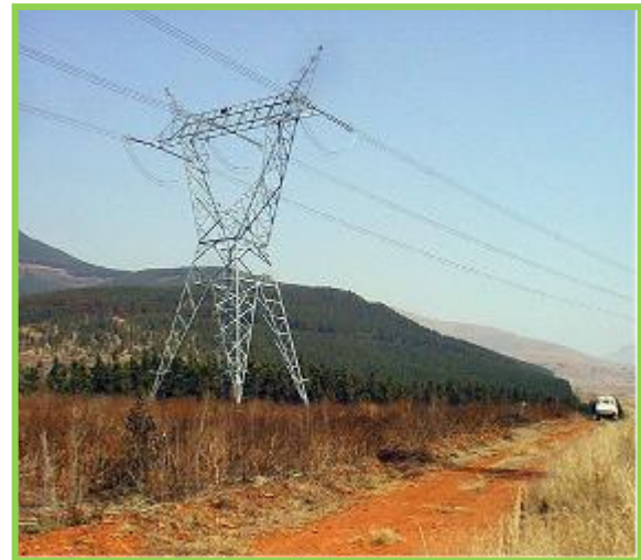
Figure 6: Photographic illustration of a Cross rope suspension tower.
