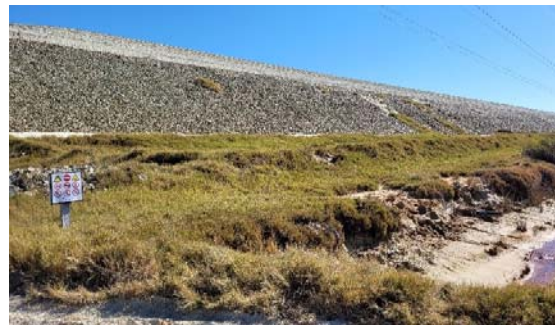
Figure 11: End point of the proposed pipelines where they will be connecting to the existing pipelines linked to the TGT 2 Tailings Storage Facility shown in the background
