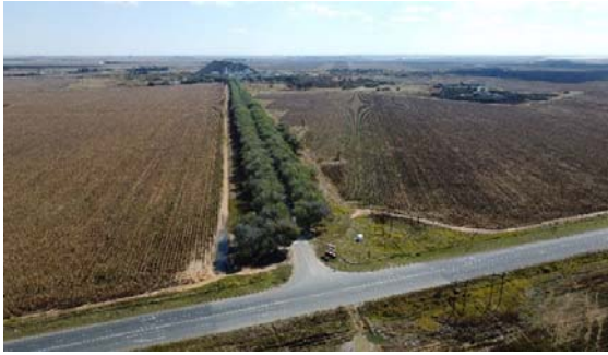
Figure 6: Picture showing the R30 where the pipeline will cross through a culvert
