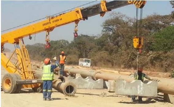
Figure 12: Example of installation of flanged steel pipeline above-ground on pre-cast concrete plinths
