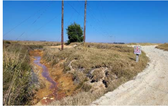
Figure 9: Picture showing the existing gravel road which is located adjacent to the proposed pipeline
