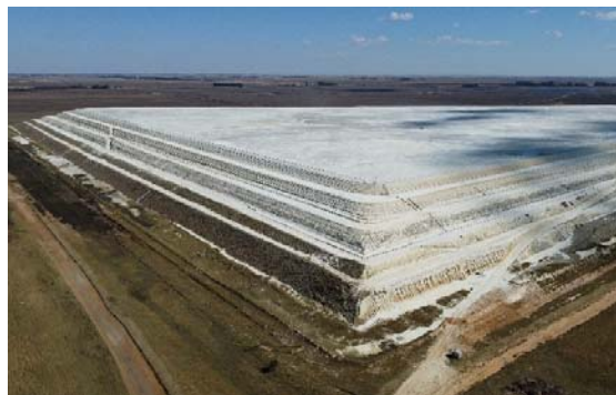
Figure 5: Tailing Storage Facility 2 which has reached their final design height and currently unserviceable
