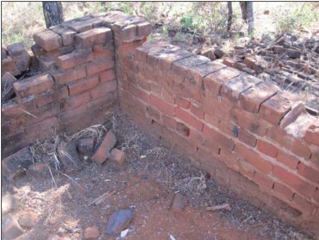
Photo 12: View of the constructed brick walls of the structure.
