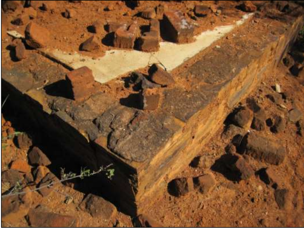
Photo 11: View of the slate stone foundations of the structure.
