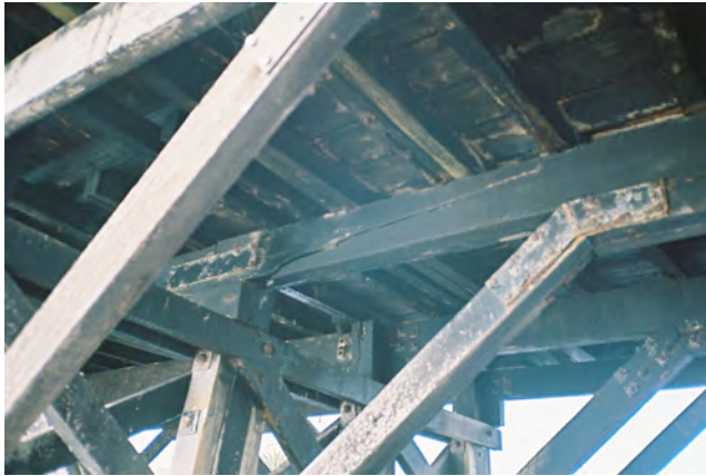
Note split beam
