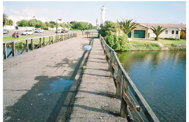
View of deck looking west
