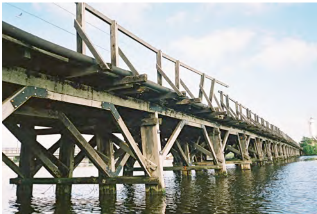
General view looking north east
