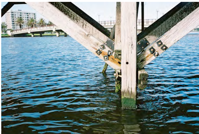
General view of lower gusset plates
