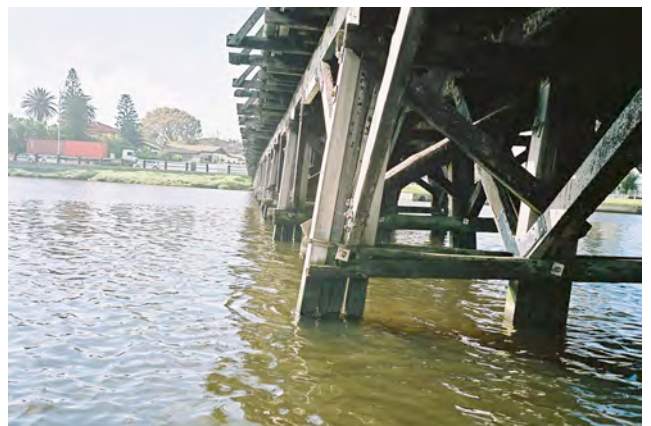
Piles still structurally in place
