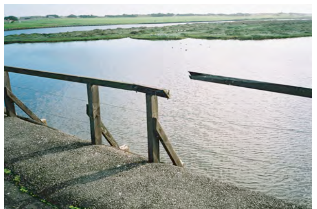
Broken handrail
