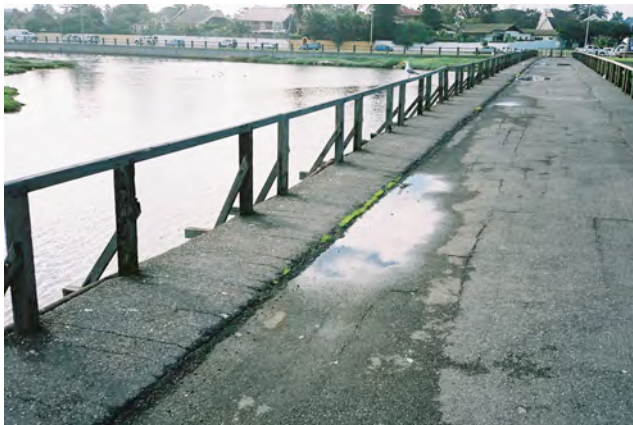
View of deck looking east
