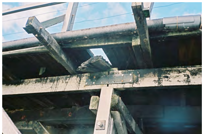
Collapsing decking
