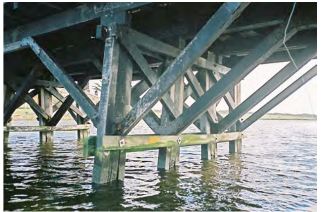
General view of bridge span
