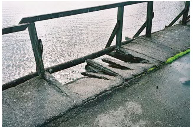
Collapsed decking
