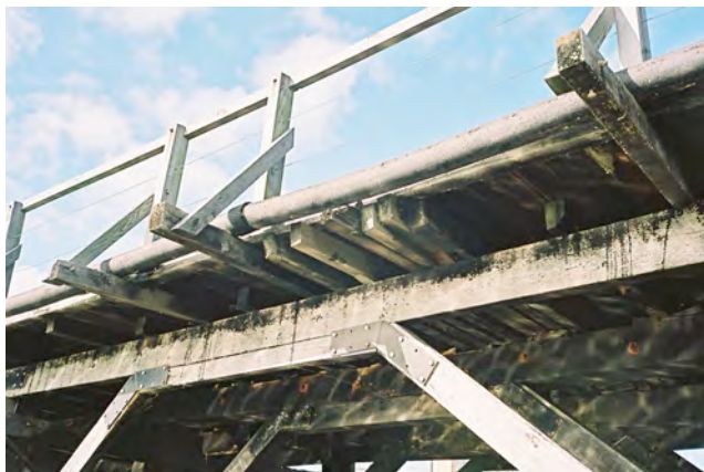
View of decking. Note packing repairs
