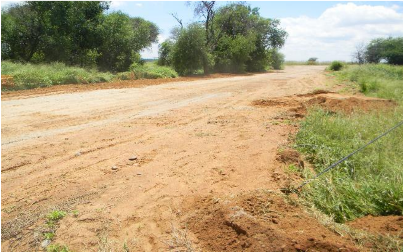
Plates 10: View of access road after rehabilitation (Author 2020)
