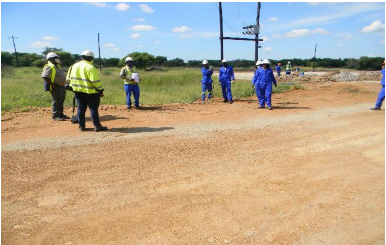
Plates 1: View of construction team during toolbox talk and briefing (Author 2021).
