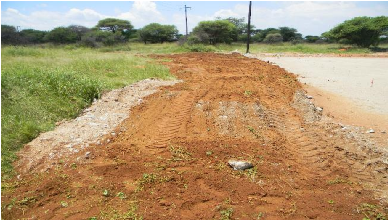
Plates 11: View of stockpiled soils rehabilitated at the site (Author 2020)
