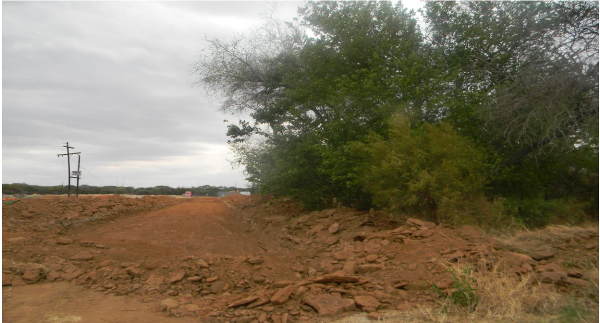
Plate 17: Shows access road under construction
